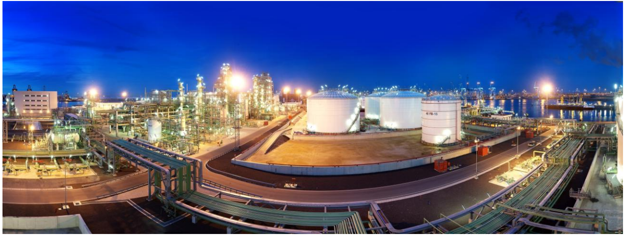
Neste Oil's renewable fuel refinery in Rotterdam in the Netherlands.
